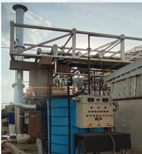
Boiler (under installation and commission) that would use Biogas as fuel at Anthem
