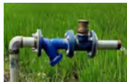
Water meters were installed in the fields to monitor water levels at SeedWorks
